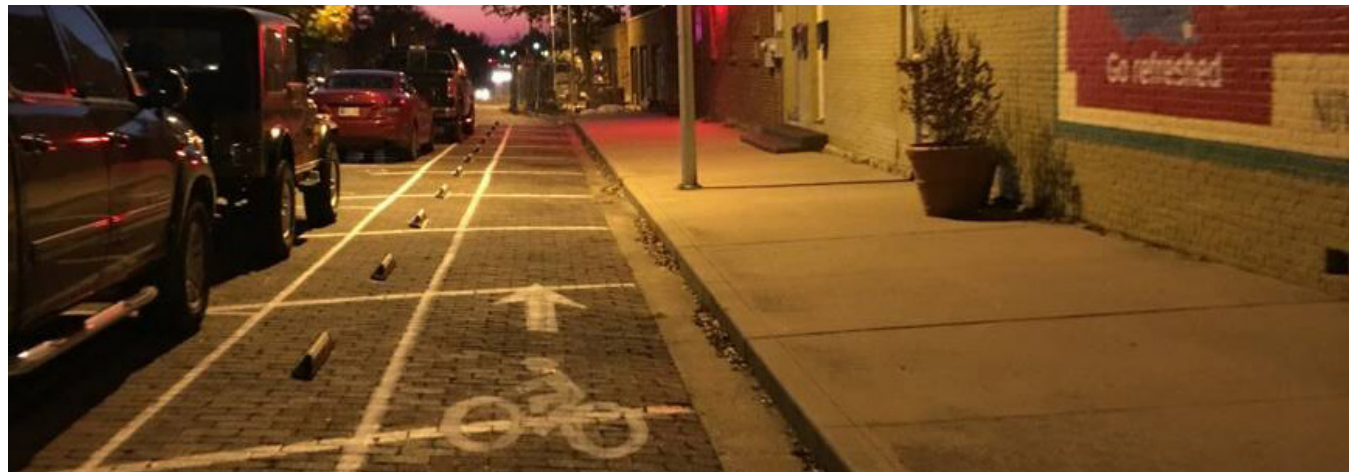
Top left: Flexible delineators were glued with Gorilla Glue on along 3rd Street (Street Plans); Top right: Armadillos are low profile and provide a great solution for locations where curbside emergency vehicle access is required. (Street Plans); Bottom: Cycle lane delineators are another low profile option for protective device, used here with a “floating” parking lane (Tim Conklin).
