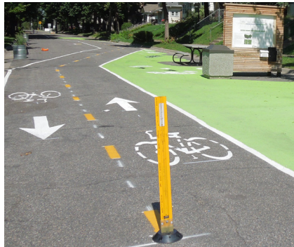
Flexible delineator - see page 28 - at the North Minneapolis Greenway pilot project (Carrie Christensen).
