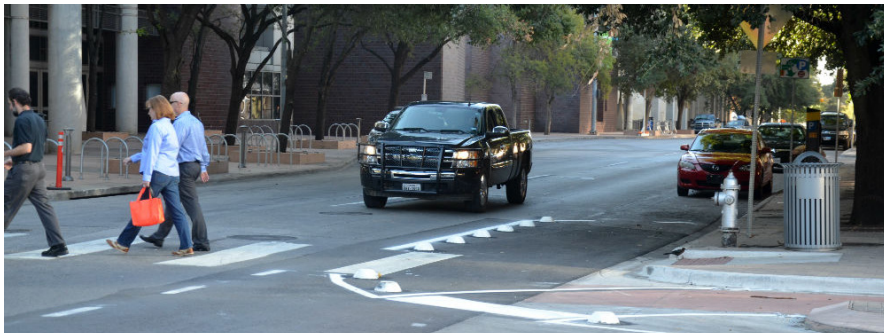
The Austin Transportation Department has used concrete buttons to create a less visually intrusive curb extension barrier. (Michael Andersen, bikeportland.org).
