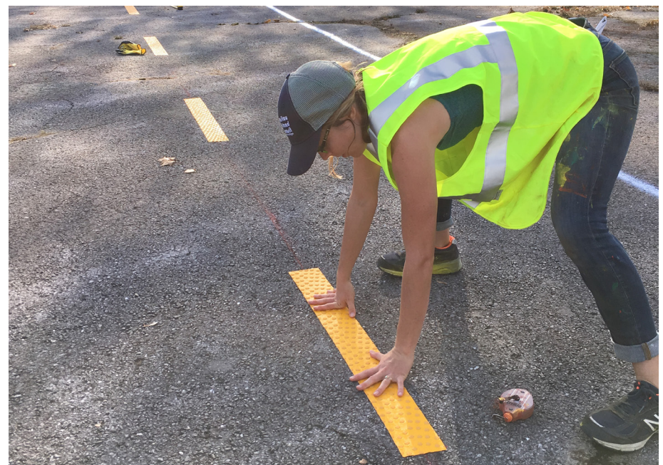
Contractor grade traffic tape is used to demarcate the center line of a monthlong protected bikeway project in Bella Vista, AR (Street Plans).
