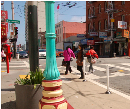
SFMTA's low-cost materials create a curb extension (Aaron Bialick, StreetsBlogSF).
