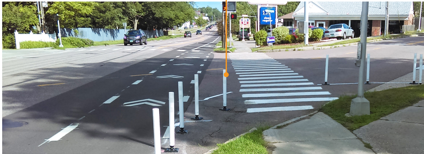
Top left: North Avenue before the pilot configuration (Google). Top right and bottom: A one-year pilot project is testing a range of pedestrian and bicycle designs / materials enhancements. (City of Burlington Public Works Department).
