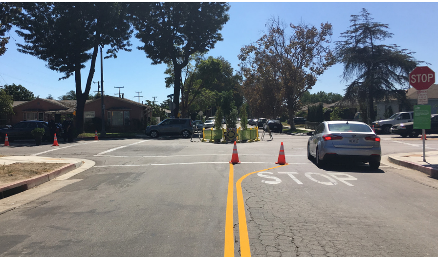
Foil-backed traffic tape is available in multiple colors, including yellow (seen here), which can be used for center line striping. Volunteers installed a very short-term splitter island with cones and yellow traffic tape to encourage people driving to navigate around a temporary mini-roundabout at the center of this Long Beach, CA intersection (Street Plans).
