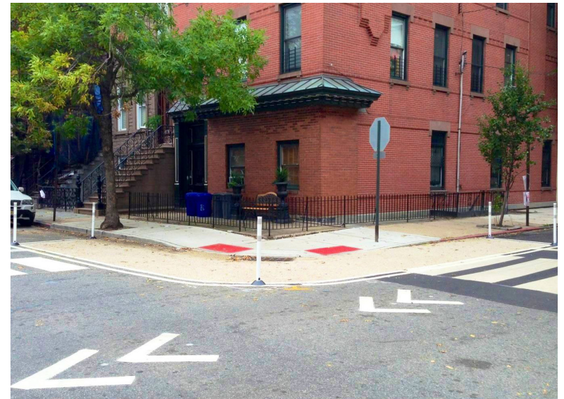
Top: Epoxy gravel used as a crosswalk surface treatment in London, England (Street Plans). Bottom: Epoxy gravel used in conjunction with flexible delineators to create a low-cost curb extension in Hoboken, NJ (City of Hoboken).
