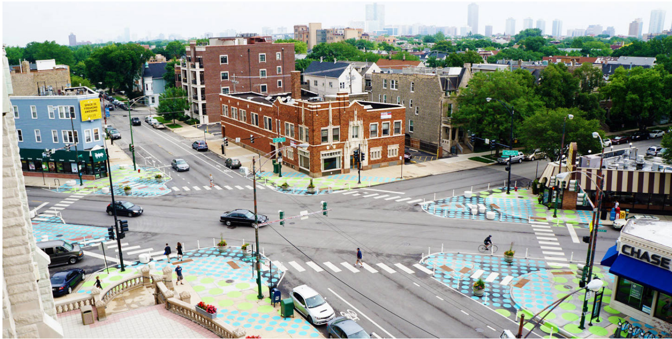
Lincoln Hub's Generous curb extensions / plazas reduce turn radii and shorten the crossing distance by 20% (Site Design Group).
