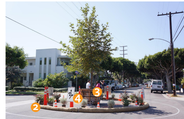
Top: A 6-month pilot traffic circle in Palo Alto, CA (Joshuah Mello); Middle: Demonstration traffic circle in Livingston, MT (Melinda Barnes, Bike Walk Montana); Bottom: Pop-up MANGO demonstration project in Santa Monica, CA (City of Santa Monica).
