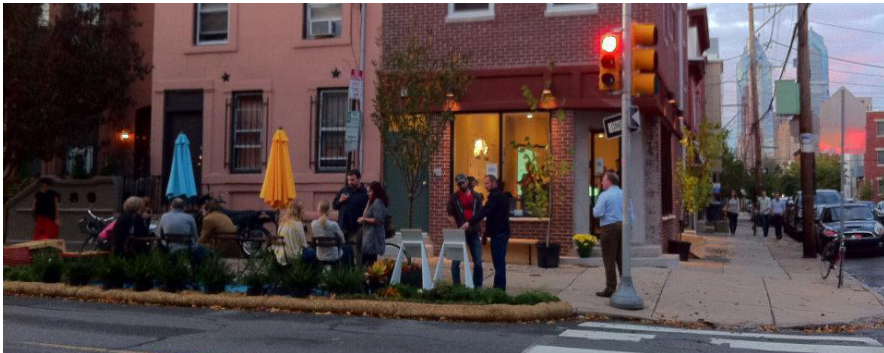
As part of the Better Block Philly demonstration projects in Philadelphia, straw wattle curbing was used to create curb extensions and expanded sidewalk space (Better Block Philly).
