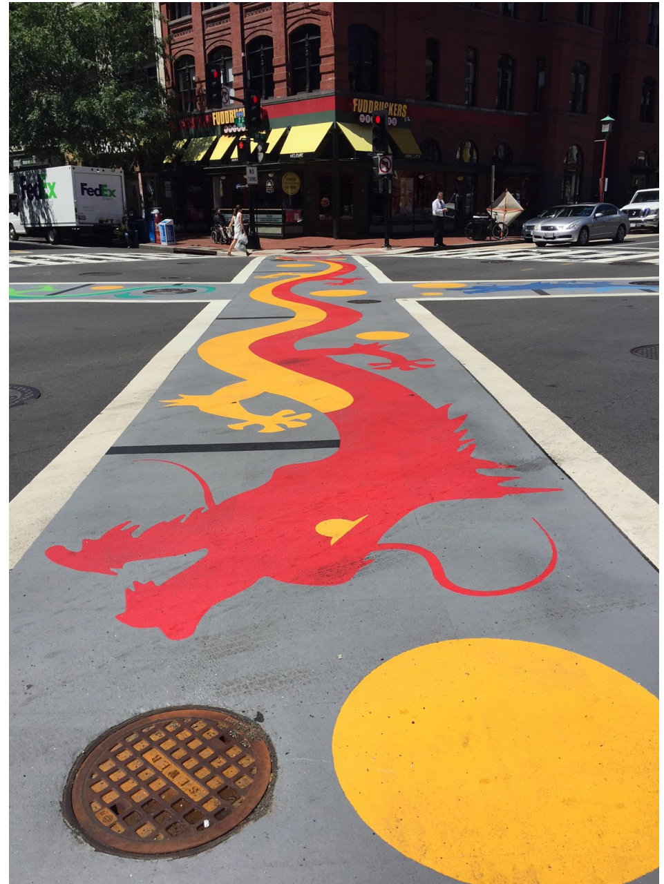
Artist Charles Bergen used Ennis-Flint's TrafficPatterns® Preformed Thermoplastic to create artistic crosswalk designs as part of the Washington, DC Chinatown Barnes Dance Public Art Project ( ennisflintamericas.com ).
