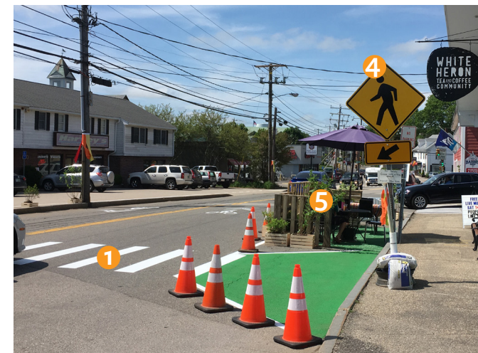
Above: A median refuge made out of straw wattle, hay bales, and flowers improve the walking (and rolling!) experience in Ponderay, ID (Street Plans). Below: A new crosswalk and curb extension improved the visibility of people walking along Portsmouth, NH’s Islington Street (Street Plans).
