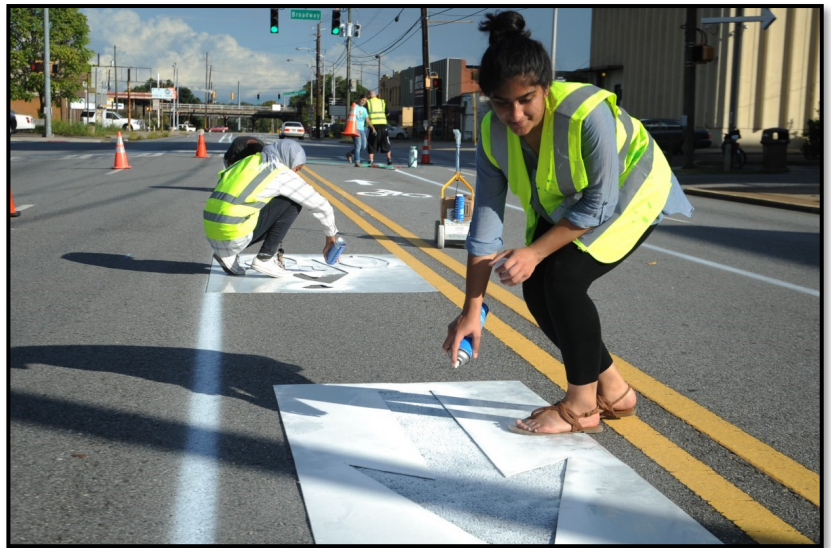
Painting bike lanes in Macon, Georgia. Source: Streetsblog USA
