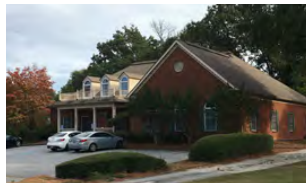
Existing medical office
