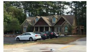
Existing medical office
