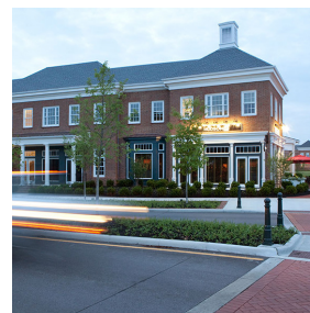
Potential future character in the southern portion of the corridor
