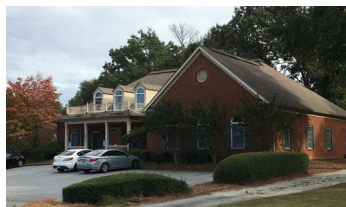
Existing medical office
