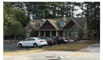
Existing medical office
